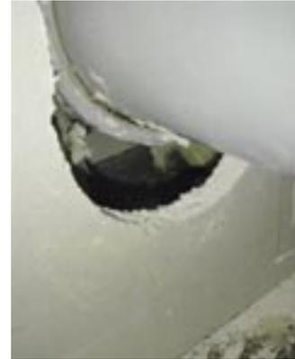
Figure 3 Gap around soil pipe at back of toilet.
