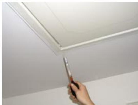
Figure 2 Air leakage through gaps around a loft hatch.
